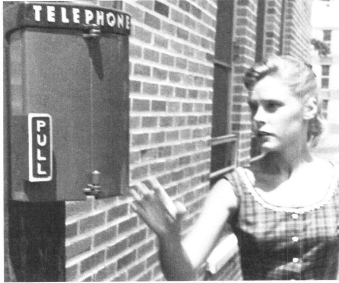
Fig. 13-77. An outdoor reporting telephone, first used in the 1950s for reporting fires, then expanded to include calls to police.
