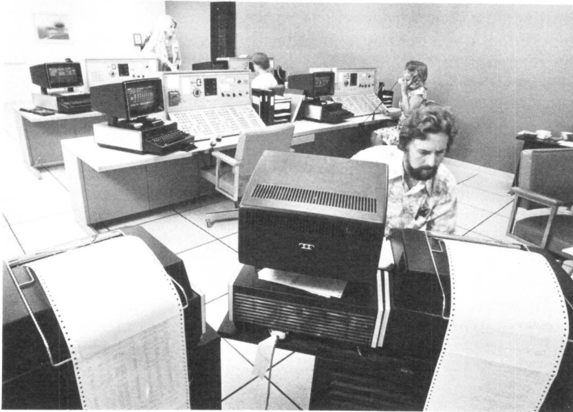
Fig. 12-8. No. 4 ESS trunk operations center in Jacksonville, Florida.
