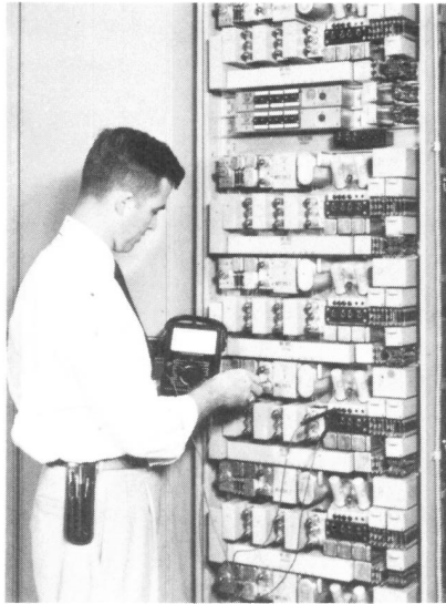
Fig. 6-5. G. Plaag adjusting one of a group of an improved version of multifrequency receivers, 1954.
