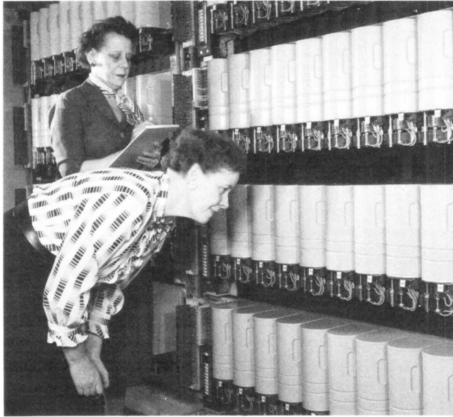
Fig. 5-12. The “switch-count” procedure for measuring usage during busy hours—visually counting the number of switches in use.
