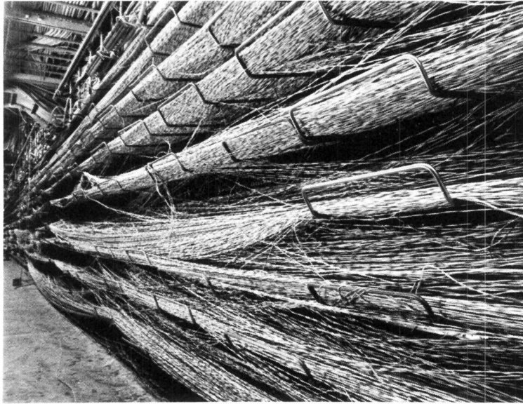
Fig. 11-37. Tangle of jumper wires on a main distributing frame—a source of trouble posing a major challenge to designers and administrators.
