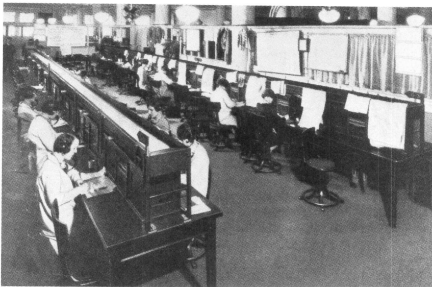
Fig. 13-68. Installation of No. 2 order turrets in the John Wanamaker department store.
