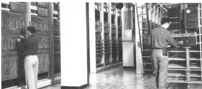
Fig. 11-22. Checking cross-connections in number group frames and AMA frames of a No. 5 crossbar-ETS.
