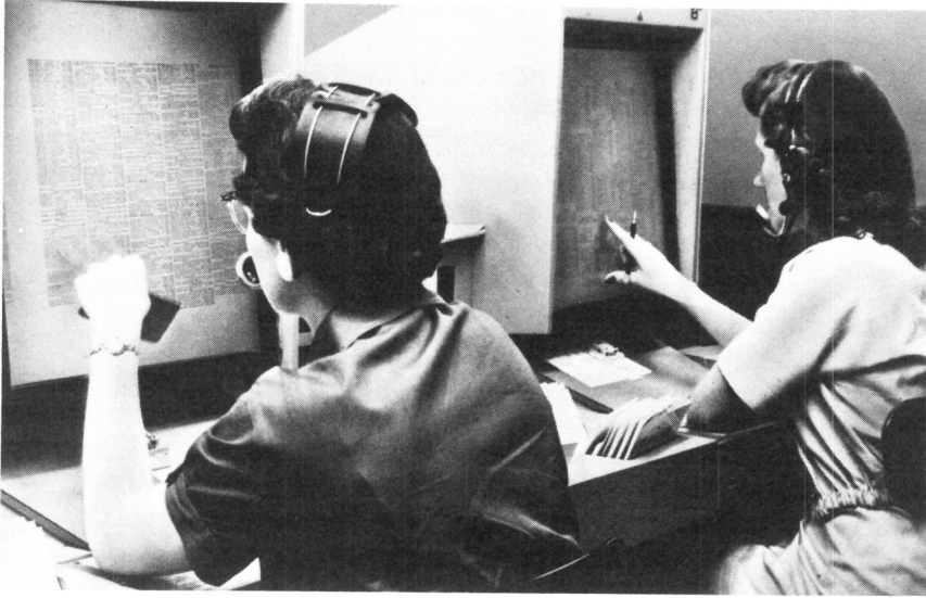
Fig. 11-28. Experimental directory assistance positions, Washington, D.C., 1958. Telephone numbers on microfilm replaced directories.
