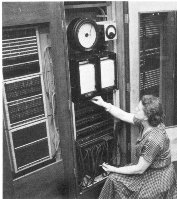
Fig. 5-15. Recording ammeters could be used for traffic-measurement, since total energy load was a measure of the number of calls in progress.
