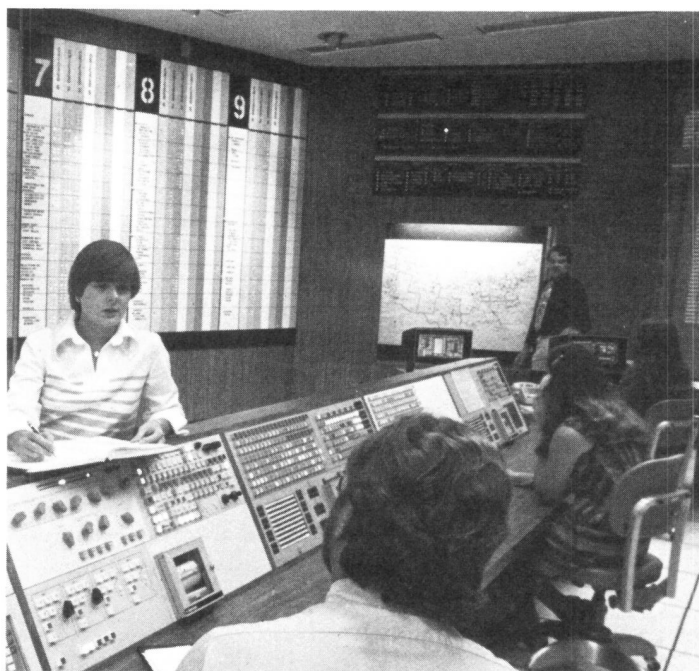
Fig. 12-4. Network management center in Chicago, Illinois where Bea Dellorto (left) checks routings with Chris Layden (foreground). Extensive network management features built into No. 4 ESS enhance ability to control traffic and avoid traffic congestion.
