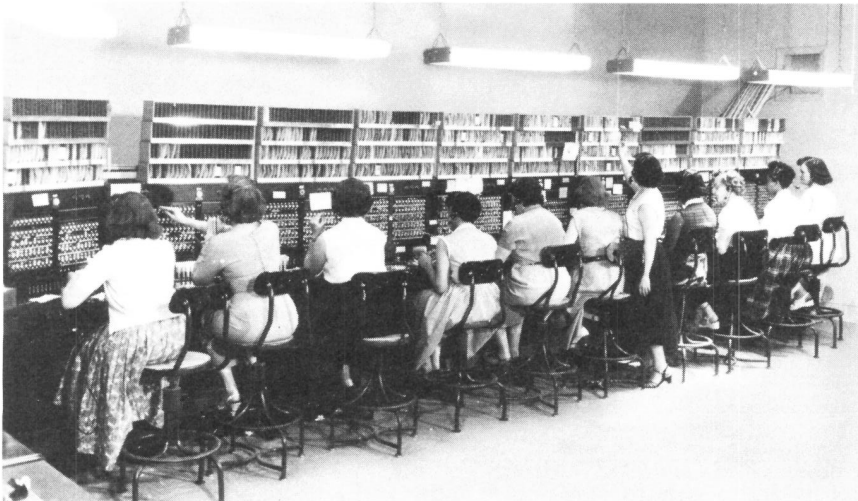
Fig. 13-64. Telephone answering service, using 557A positions developed in 1955.
