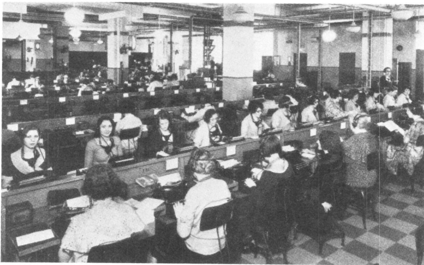
Fig. 13-70. Western Union installation of No. 3 order turrets, developed in 1932. The No. 3 was the first turret with automatic call distributing and call sequencing.
