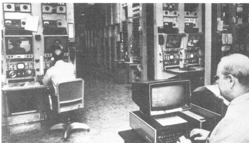
Fig. 13-91. Automatic switching and surveillance of television network transmission in 1978.
