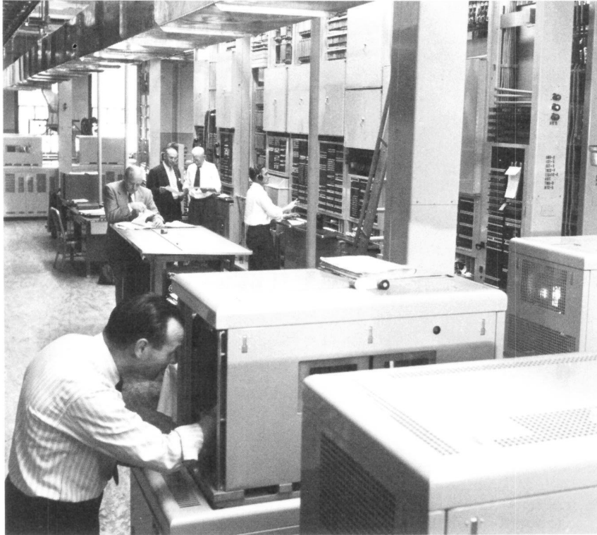
Laboratory installation of card translators, about 1952. A key system element in the growth of nationwide dialing by customers, the card translator interpreted the six digits of the area code and office code of a called telephone number. These digits caused one metal card to drop down from a stack of about 1000 cards. According to which holes in the cards were or were not enlarged, light passed through to photo-detectors to specify the information needed to select a route for a long distance call.
