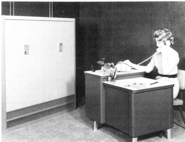
Fig. 13-15. Attendant controlling an initial 101 ESS switch unit (left), which serves up to 200 telephone lines.
