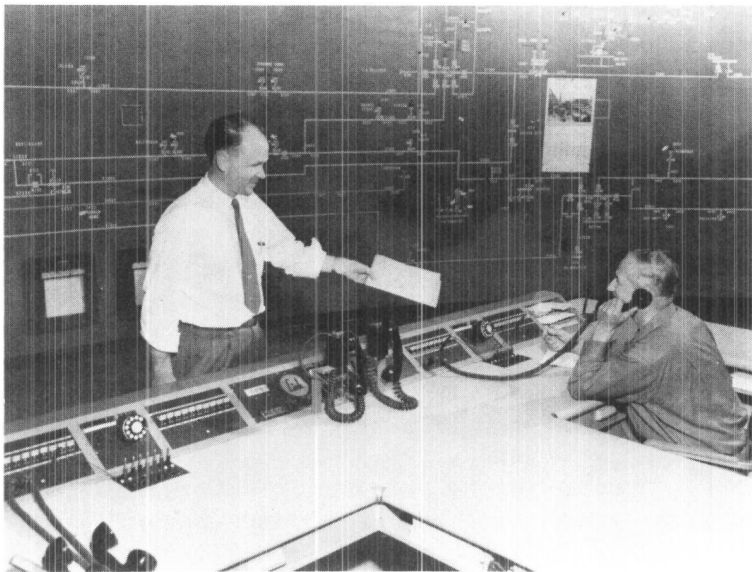
Fig. 13-76. Typical 508 PBX installation, developed in the early 1950s to meet the special requirements of utilities, railroads, pipeline operations, and similar markets needing dispatching services.
