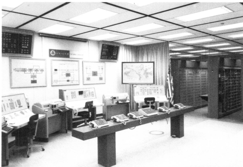
Fig. 9-46. Part of the UNICOM test model—switching center consoles and digital and analog station control sets.
