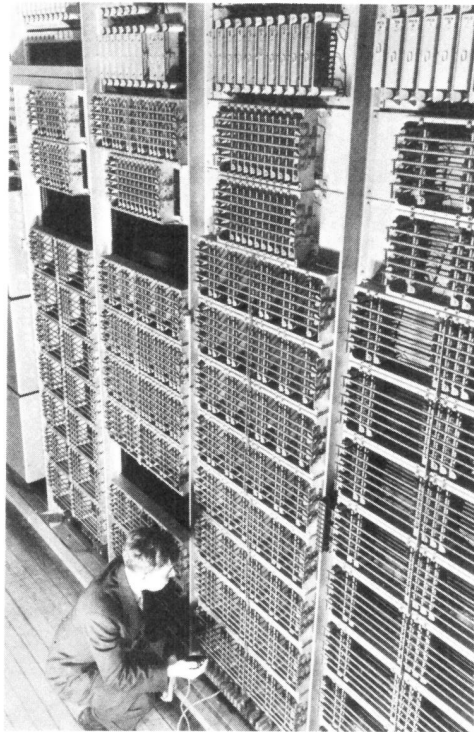
Fig. 4-3. Bell Labs experimental crossbar switching equipment, early in the 1930s.
